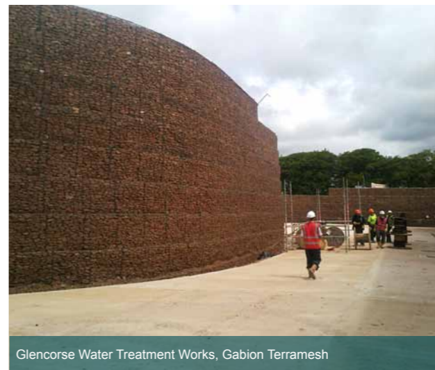
Glencorse Water Treatment Works, Gabions
