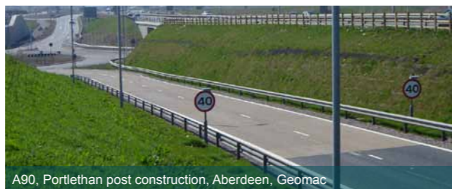
A90, Portlethan post construction, Aberdeen, Geomac
