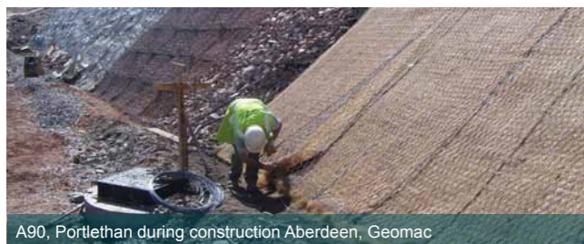
A90, Portlethan during construction Aberdeen, Geomac
