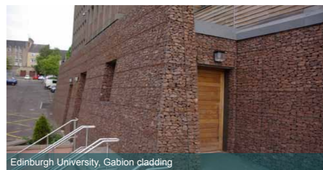
Edinburgh University, Gabion cladding
