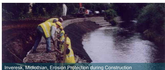
Inveresk, Midlothian, Erosion Protection during Construction
