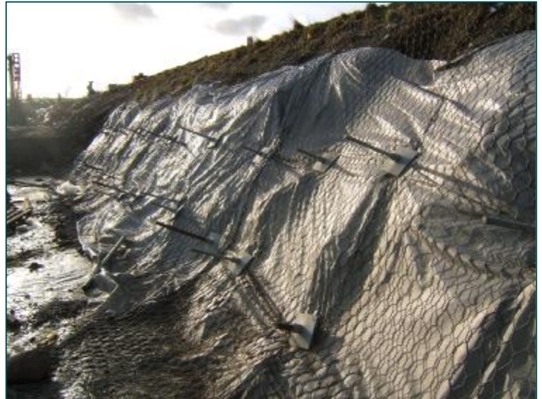
Before Maccaferri Commenced Construction
