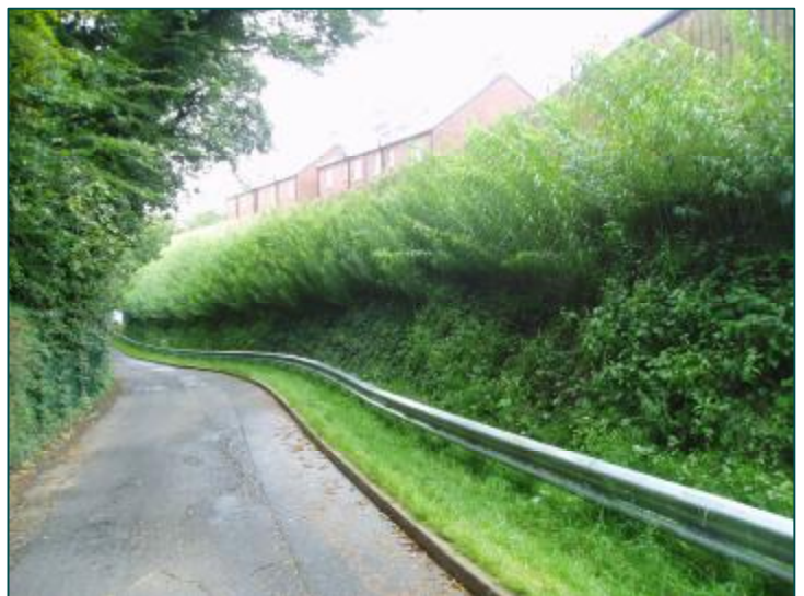
Project two years after completion
