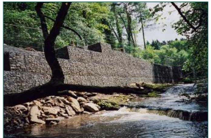
Gabion Retaining Wall - Balerno, Scotland
