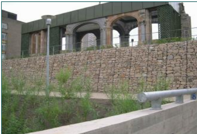
Gabion Retaining Wall - former Rotten Row Hospital, Central Glasgow.
