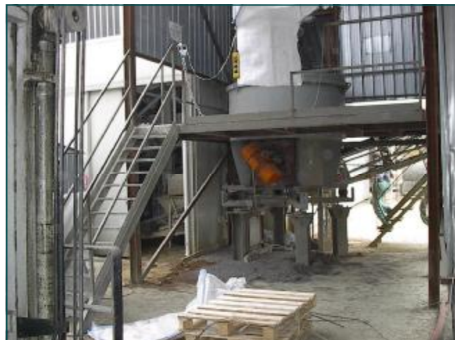
Maccaferri Doso machine installed at the batching plant
