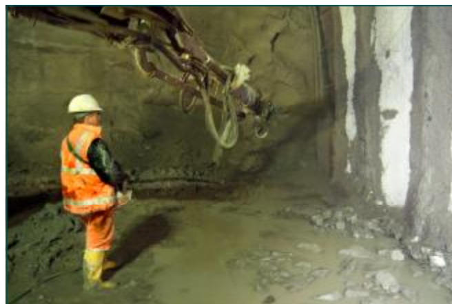
Sprayed concrete primary lining with fibre reinforcement
