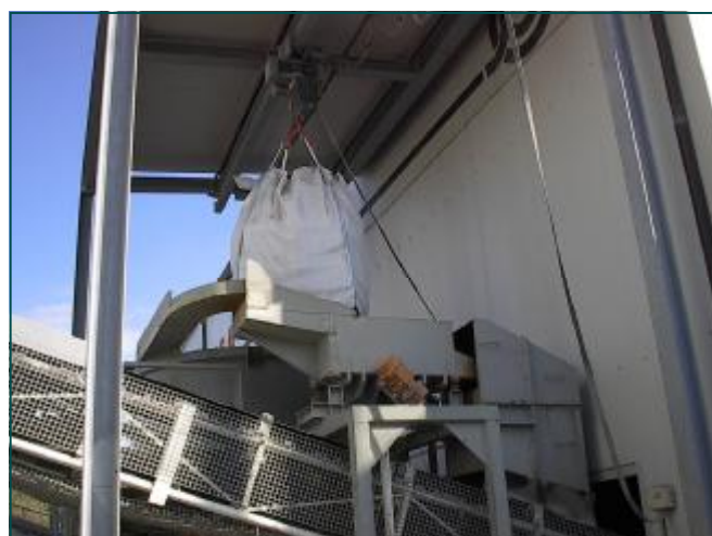
Loading Wirand® fibres into the dosing machine
