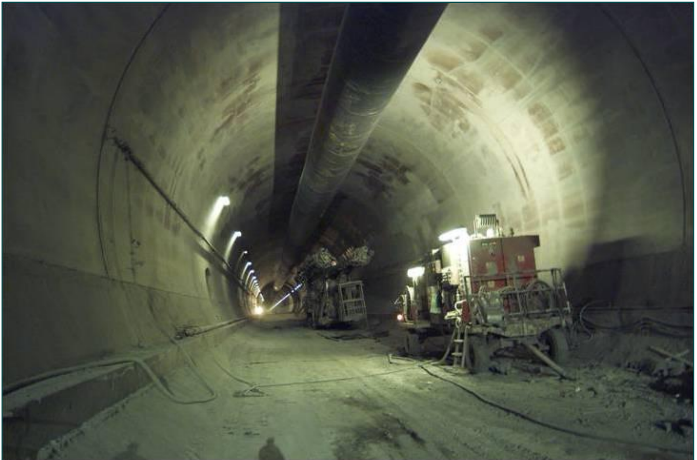
View of the completed tunnel awaiting track laying
