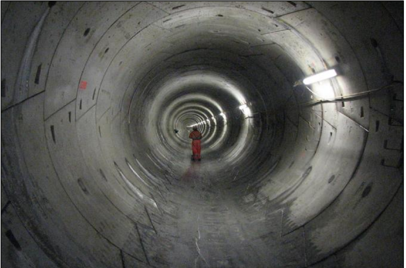
View of the completed tunnel showing installed precast segments
