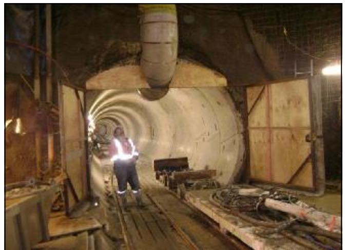
View of tunnel from the access shaft
