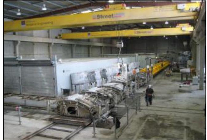
Wilson Tunnelling precasting facility
