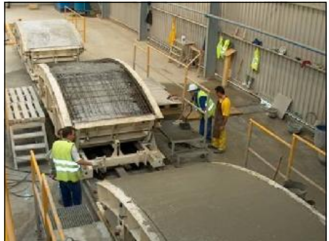
Filling segment moulds
