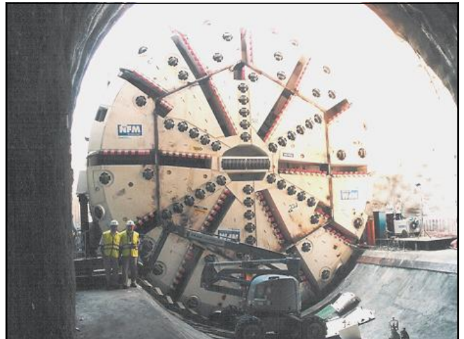
View of TBM at tunnel mouth
