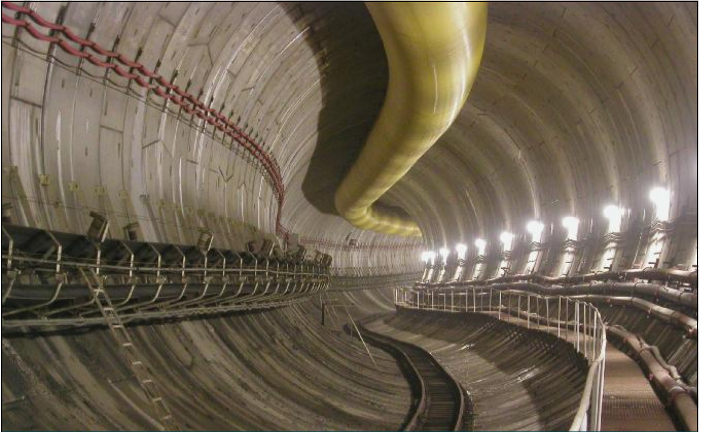
Tunnel heating completion, awaiting track laying
