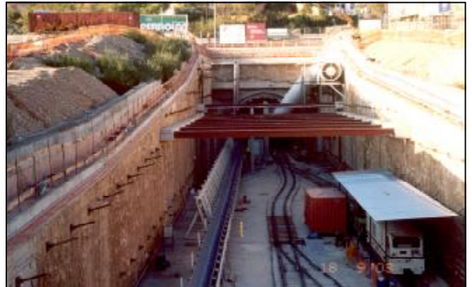
View of tunnel portal
