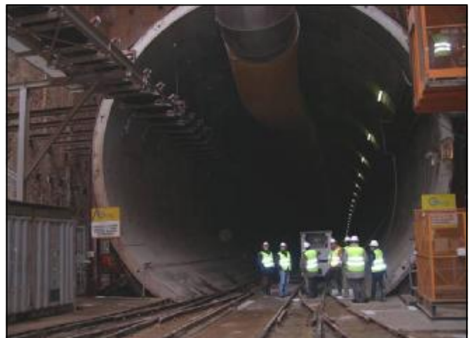
Tunnel portal showing diameter of tunnel
