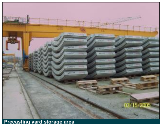
Precasting yard storage area
