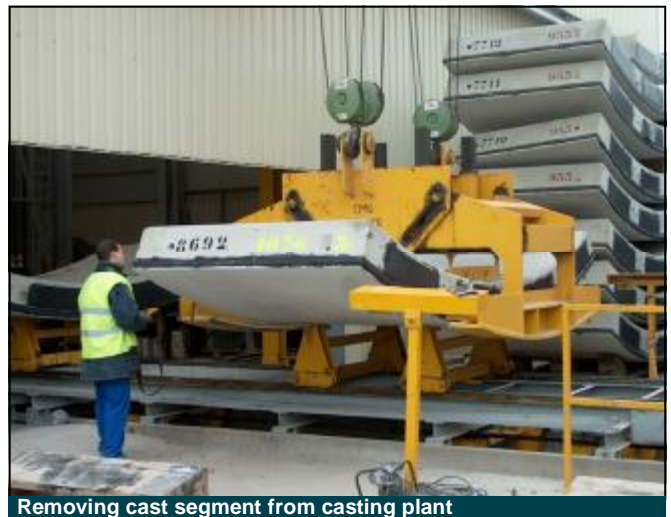
Removing cast segment from casting plant
