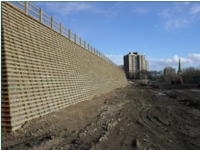
Loadman Street, Newcastle - Immediately after Construction
