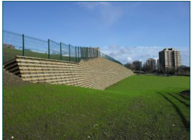
Loadman Street, Newcastle after Site Completion
