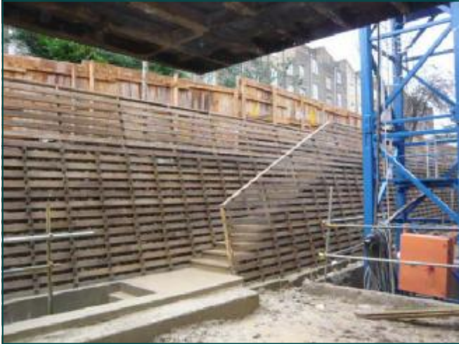
Access Steps incorporated into a Timber Crib Wall
