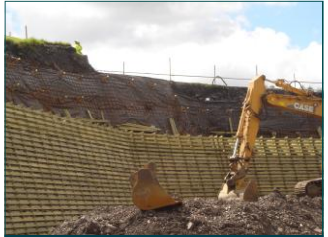
Timber Crib fascia to a soil nailed slope - During Construction
