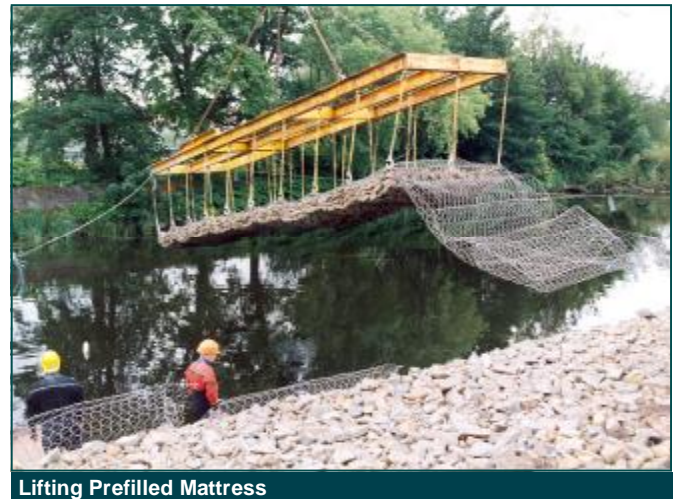
Prefilled Gabions at toe of railway embankment
