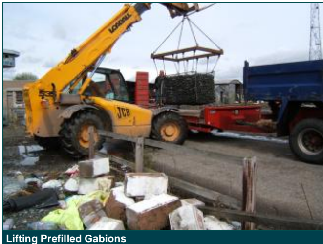
Installing Prefilled Gabions
