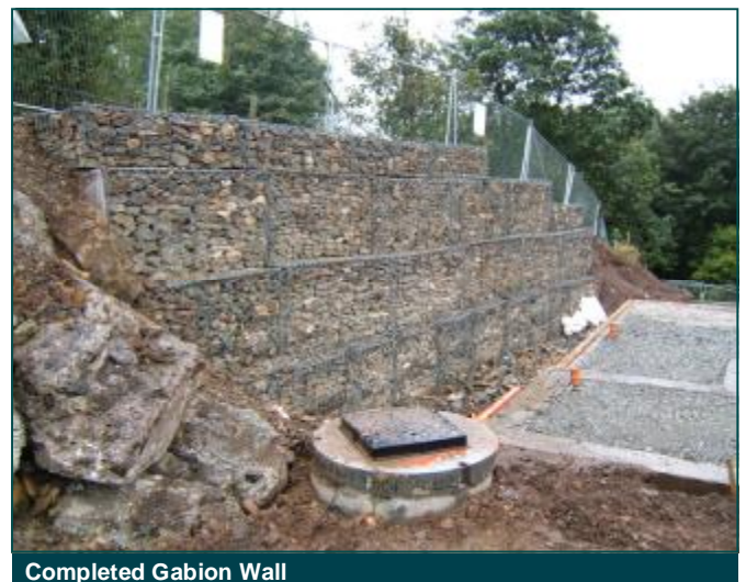
Completed Gabion Wall
