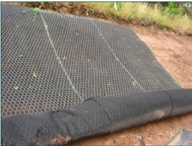
During Construction - MacMat® R
