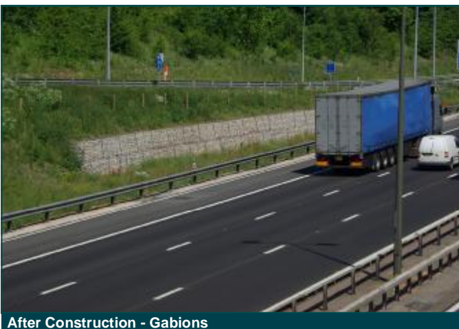
After Construction - Gabions
