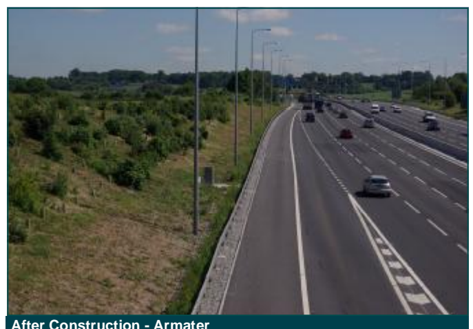
After Construction - Armater
