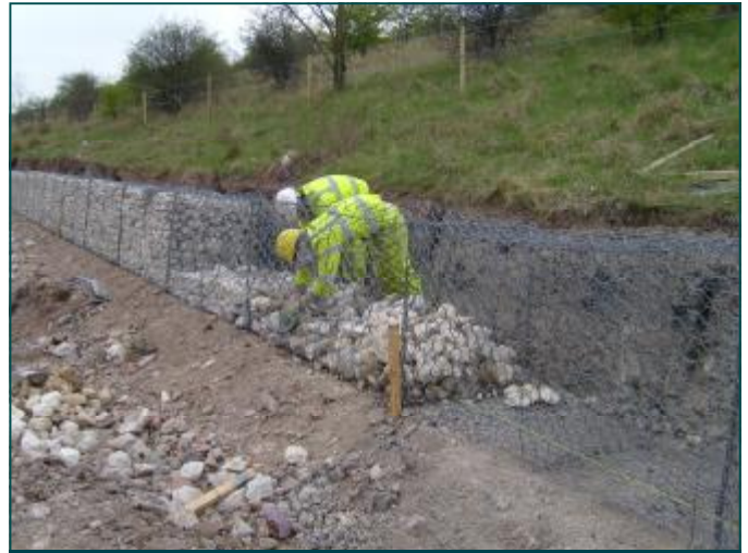
Hand placing the stone in the gabion baskets
