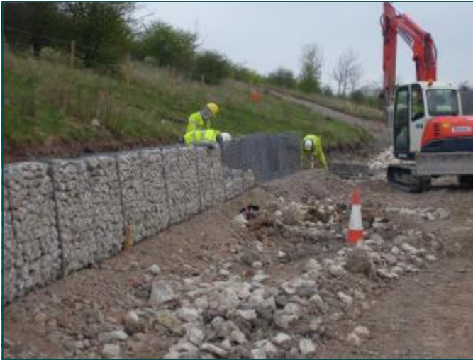
During Construction - 80m long, 1m high
