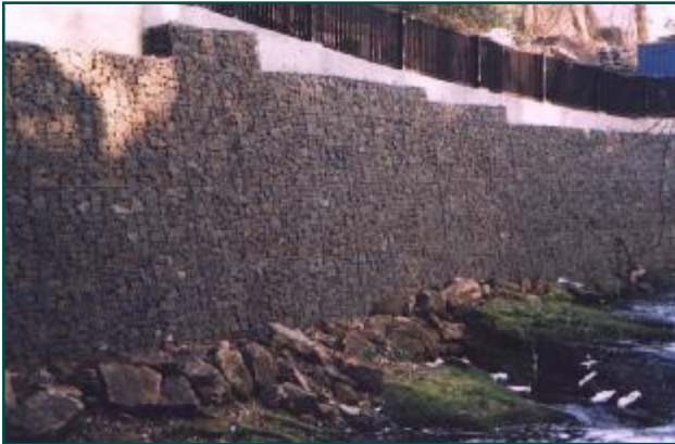
Immediately Post Construction, Balerno
