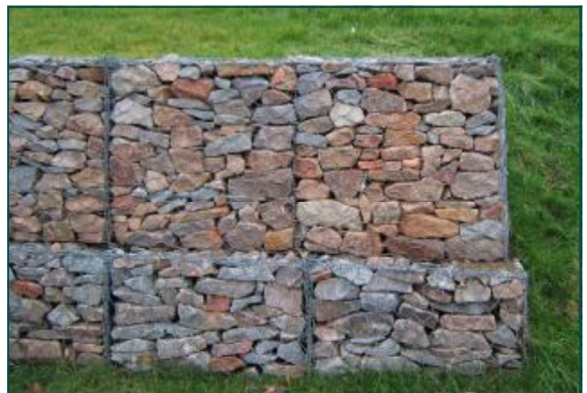
After Completion - Woven Gabions
