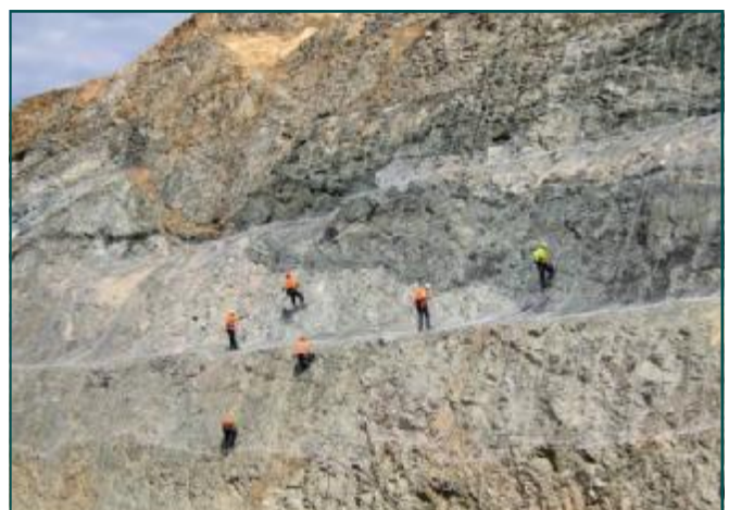
High strength Steelgrid being installed on rockface
