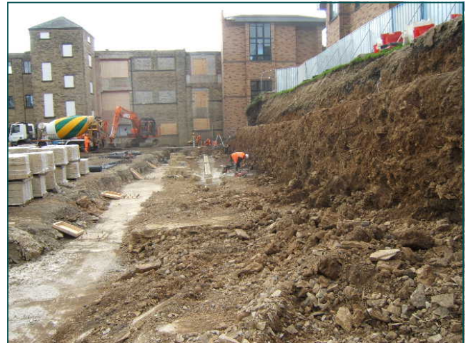
Excavation ready for MacWall against 'rock-face' at right
