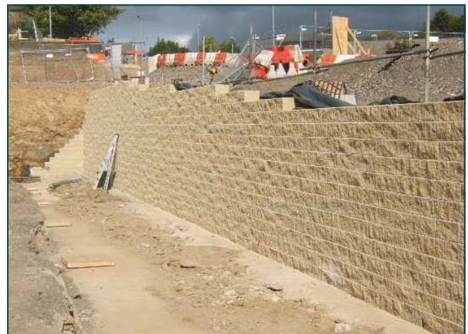
Nearing full height of wall
