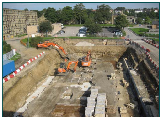
View of site, showing excavation to be retained
