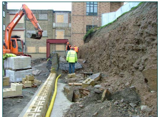
Early construction at foundation level; note drainage pipe
