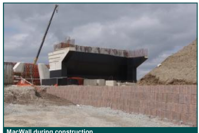
MacWall during construction
