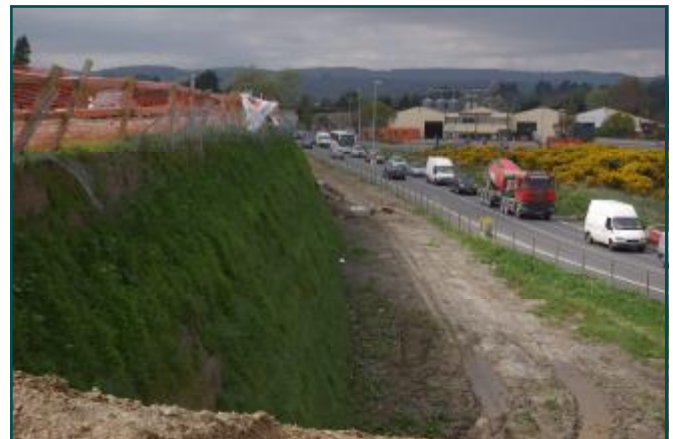
Green Terramesh reinforced slope under construction
