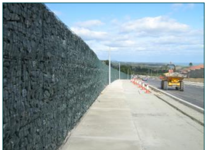
Gabion retaining wall on project
