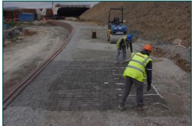
Installing Enkagrid PRO geogrid reinforcement to wall
