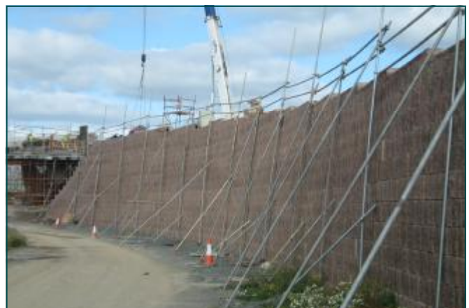
During construction of MacWall
