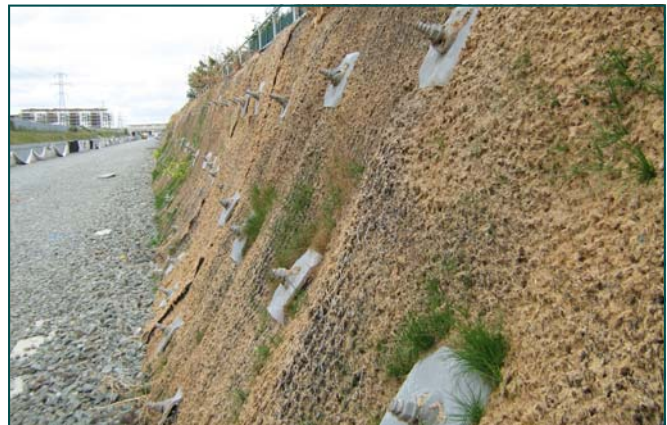
MacMat R and Soil nails after hydroseeding
