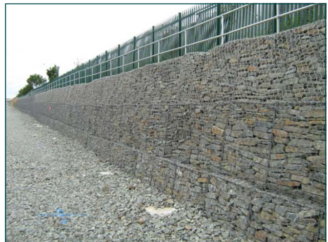
Gabion installation
