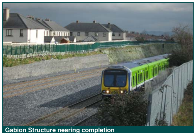
Gabion Structure nearing completion
