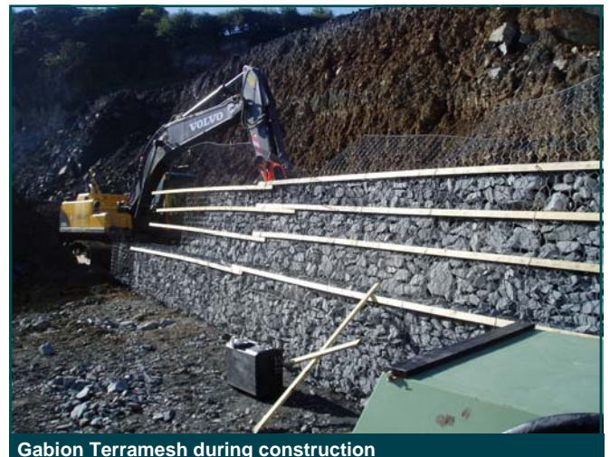
Gabion Terramesh during construction
