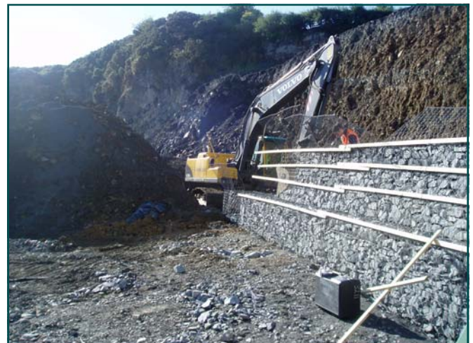
Gabion Terramesh during construction
