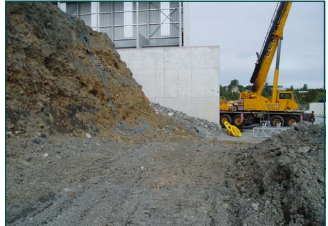
Before construction. Note aggregate hoppers in background.
