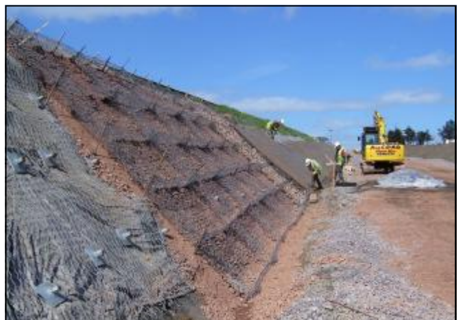
Geomac during installation
