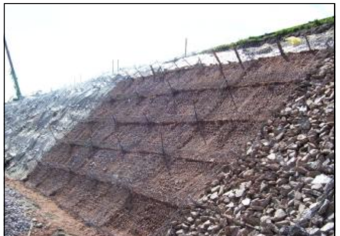
Geomac during installation showing partially filled units
