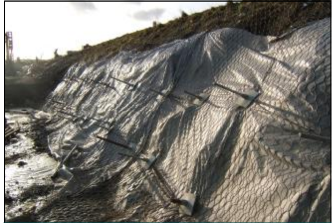
Empty Geomacs, placed on soil-nailed slope
