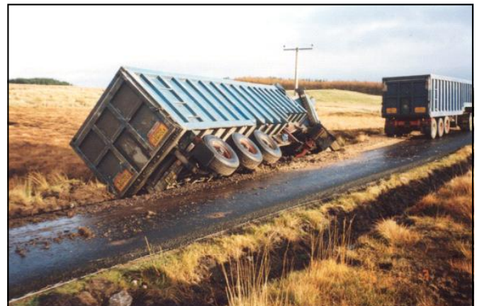
A tipper truck falls off the Floating Road with dramatic results
