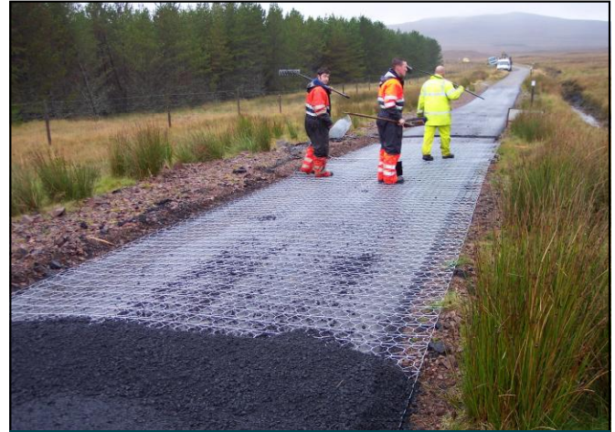
The B873 reconstructed with RoadMesh
