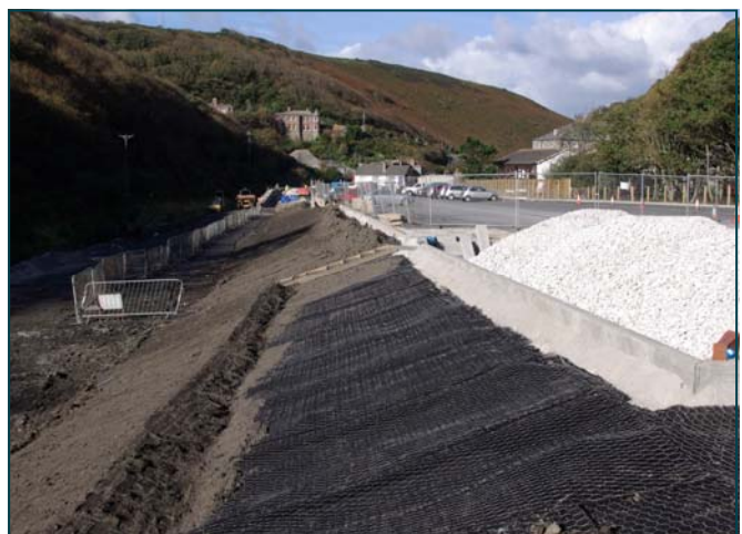
MacMat-R lids, prior to being covered in top soil
