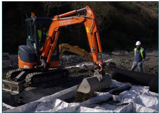
Filling the Reno Mattresses with site won material
