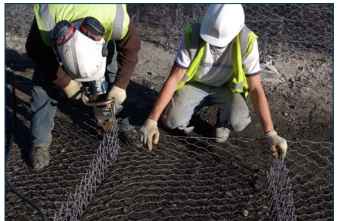
Construction of the Reno Mattresses
