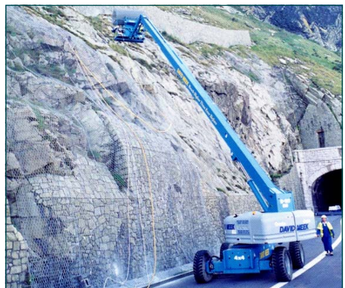
Rockfall protection netting during construction
