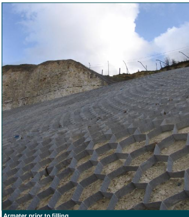
Armater prior to filling
