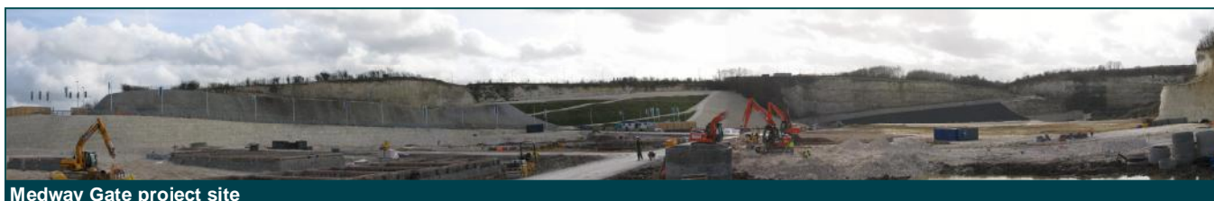
Medway Gate project site
