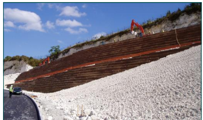
Green Terramesh during construction
