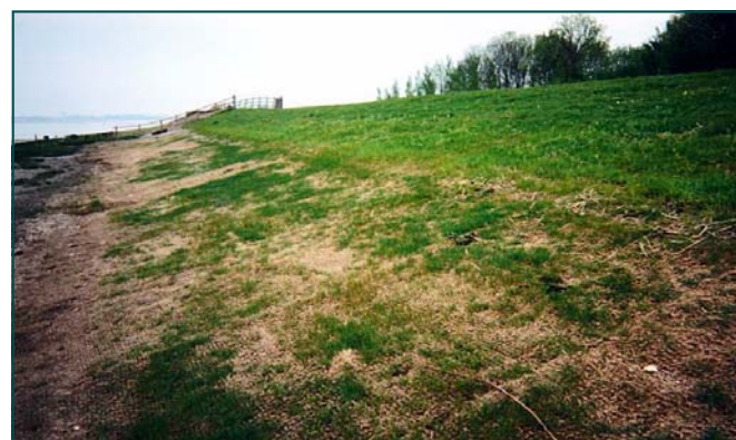
Reinstated bank and grass seeded
