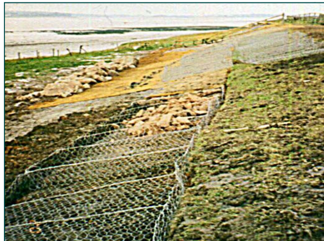
Erosion scour trimmed and Geomacs in place
