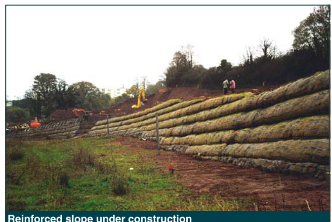
Reinforced slope under construction
