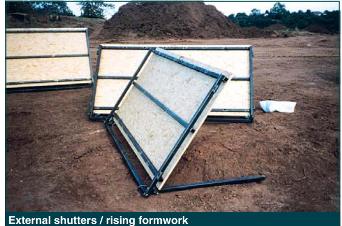
External shutters / rising formwork
