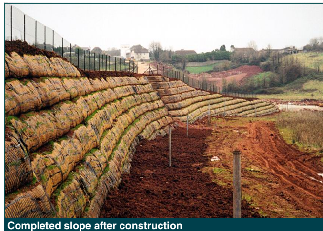
Completed slope after construction
