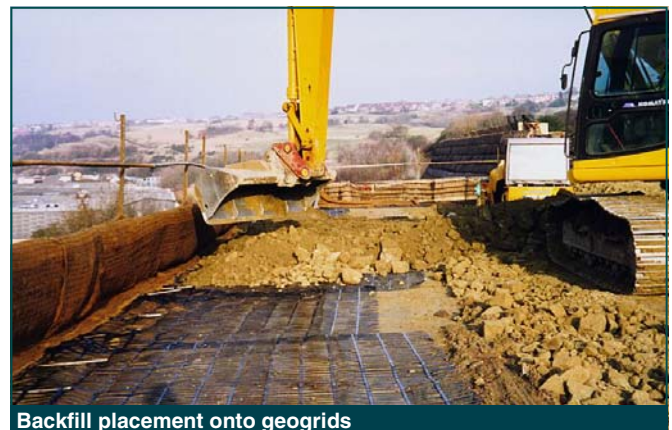
Backfill placement onto geogrids
