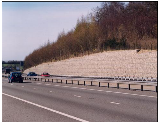
Post construction, North bound off-slip
