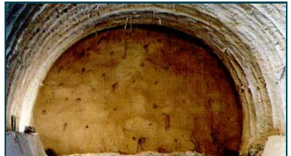
Fig. 3 - Typical sprayed fibre application using Wirand
