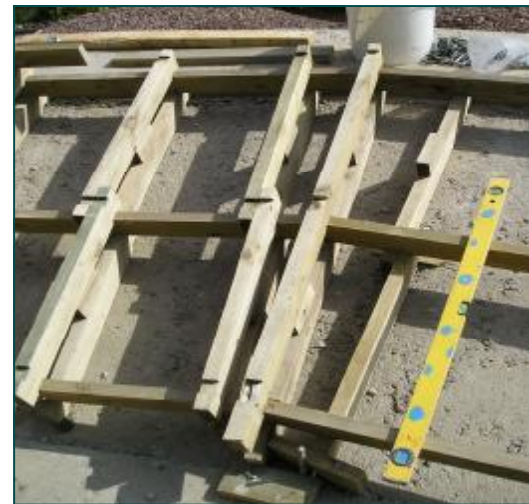
First courses of crib units at a corner of the structure
