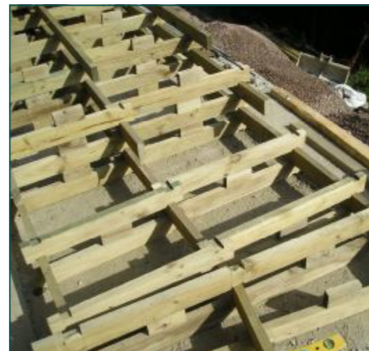
Note the bearing blocks between header units, used on taller structures
