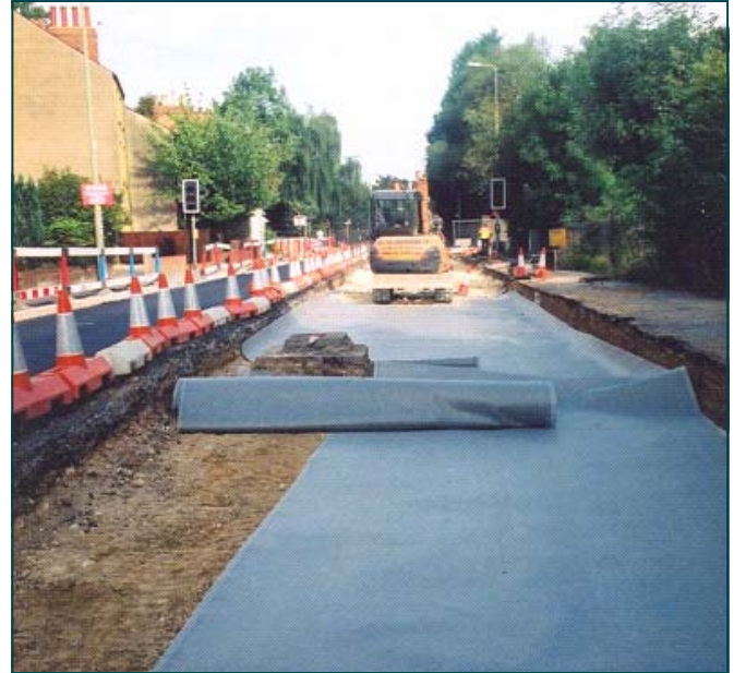
Enkagrid TRC during installation
