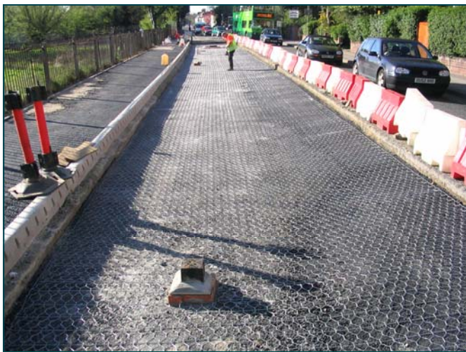
RoadMesh during installation
