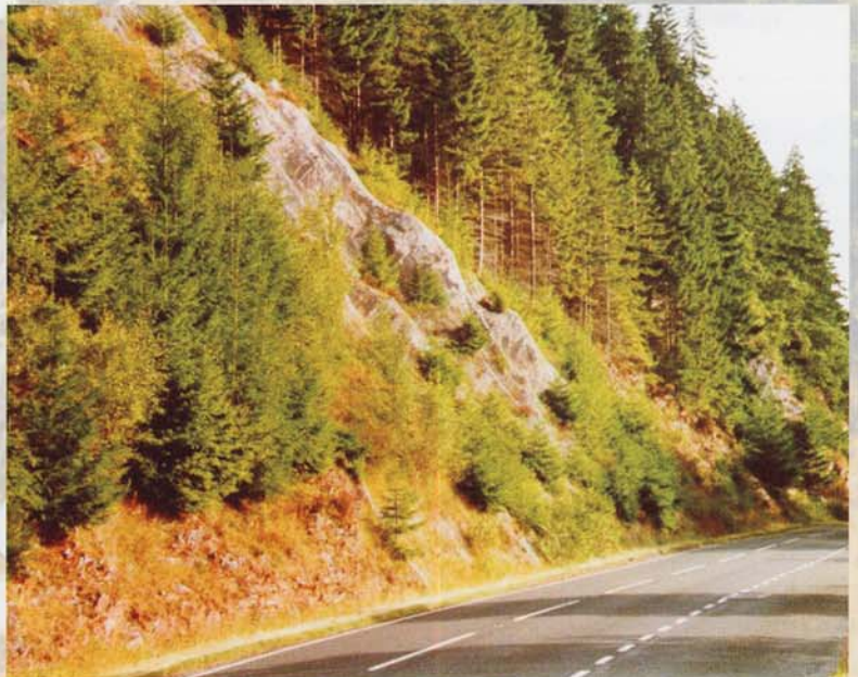
Figure 1 - Vegetated Rockfall Netting Installation A82, Loch Ness, Scotland
